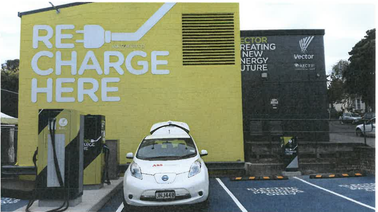
Electric vehicle charger station installation at Newmarket Substation, Gillies Ave
