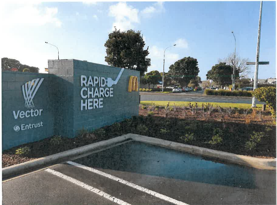
Electric vehicle charger station installation at McDonalds, Greenlane
