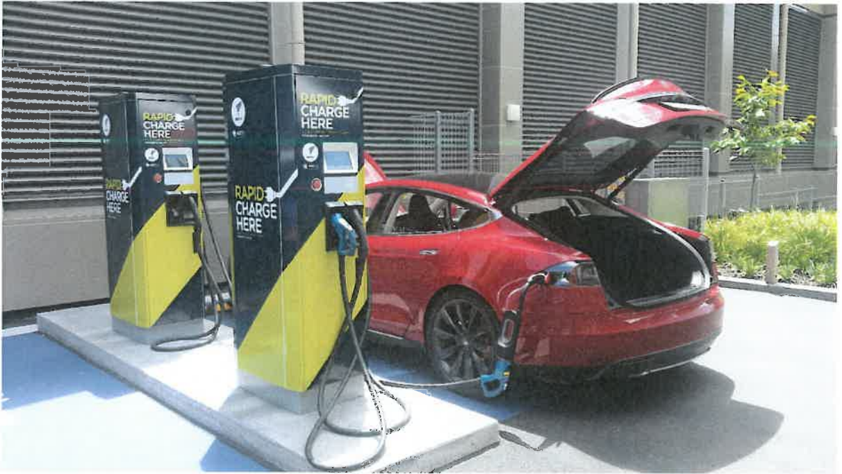
Electric vehicle charger station installation at Hobson Substation, Hobson Street
